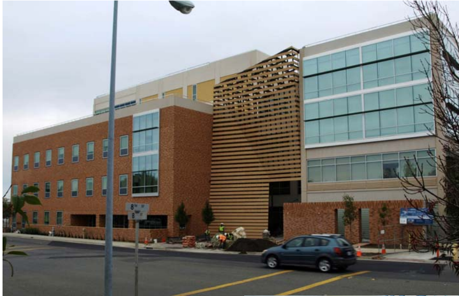
Leo J. Trombatore State Office Building Caltrans District 3 Marysville, CA
