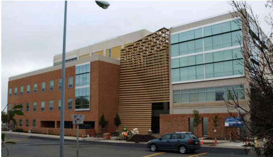
Leo J. Trombatore State Office Building Caltrans District 3 Marysville, CA
